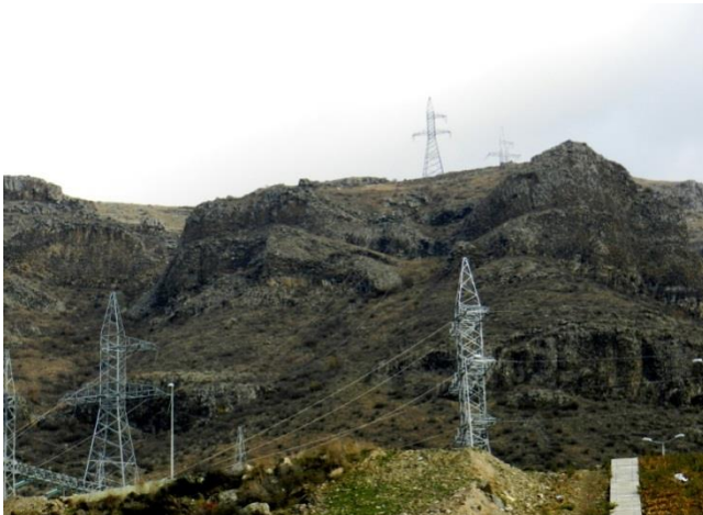
Figure 1. . Towers near the Paravani substation
