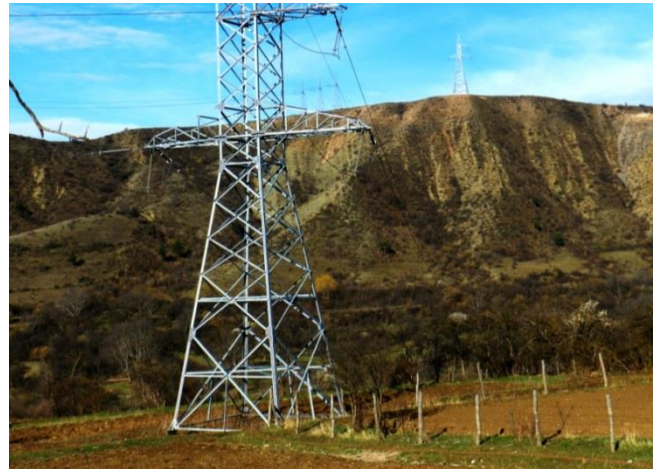
Figure 2. Tower in the crossing of the Tsinubnistskali gorge
