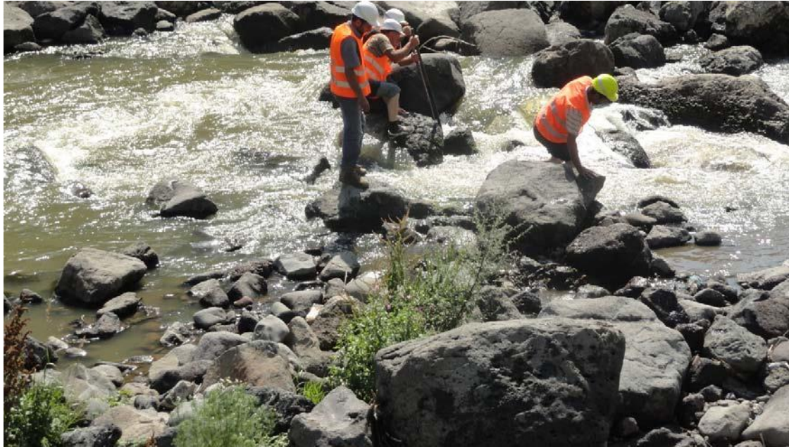
On the basis of the recommendation, to free the riverbed from the big boulders is taking place.
