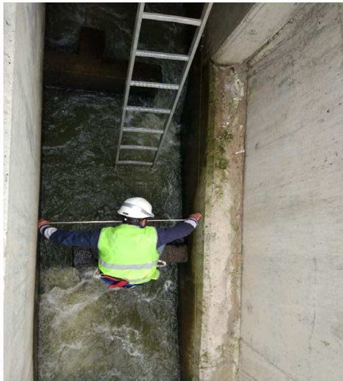
Preparatory Works for Installation Fish Trap in the Fish Passage
