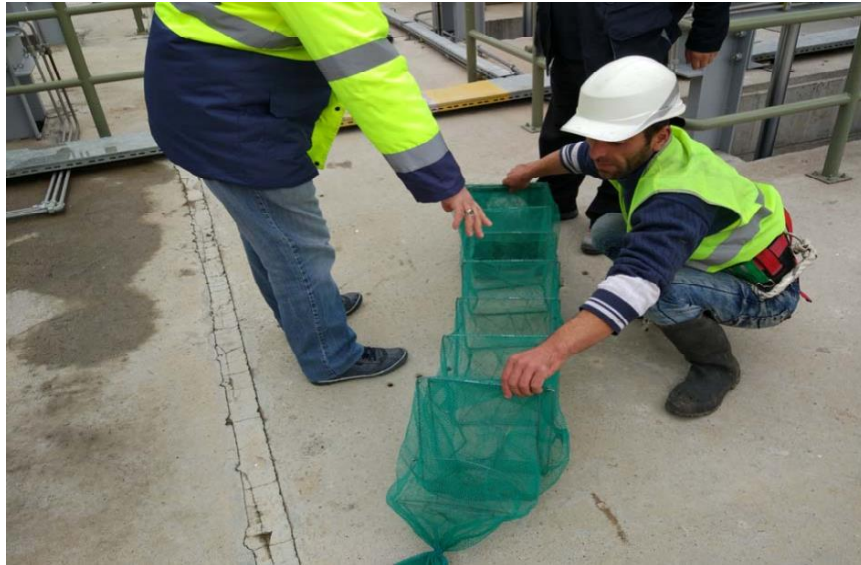
Preparing Fish Trap for Installation in the Fish Passage
