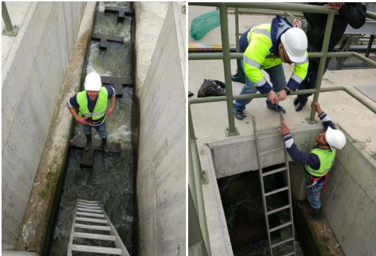
Preparatory Works for Installation Fish Traps in the Fish Passage
